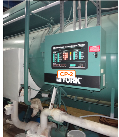
West Side View
