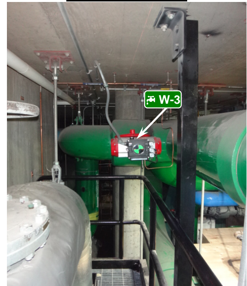
North Side View
