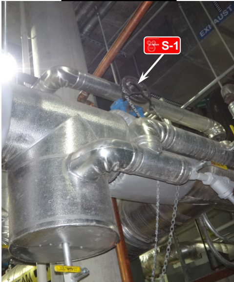
West Side View
