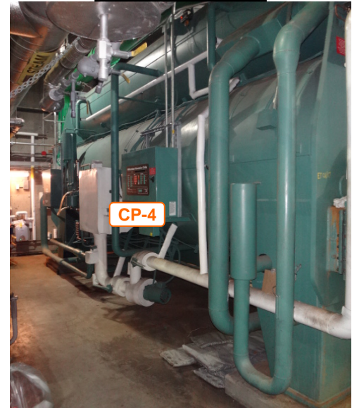
North Side View
