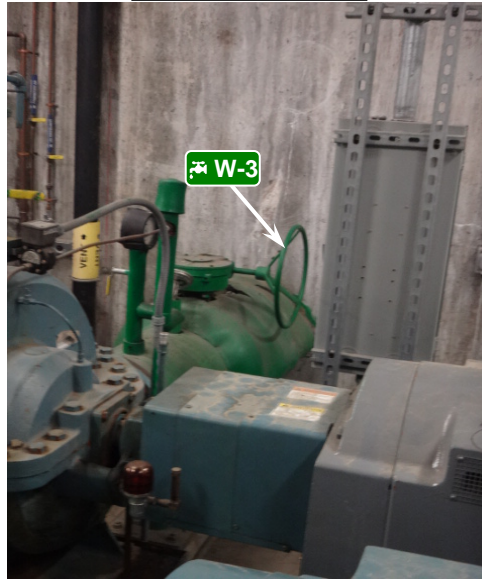
West Side View
