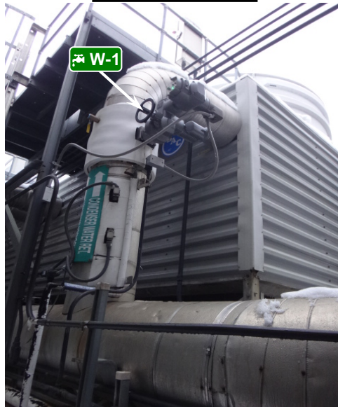
West Side View
