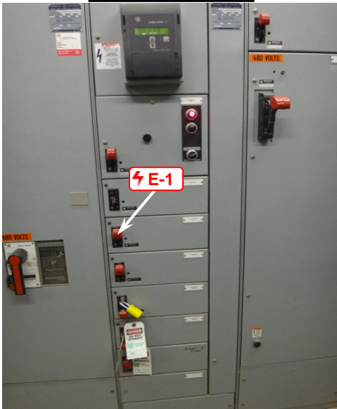
West Side View
