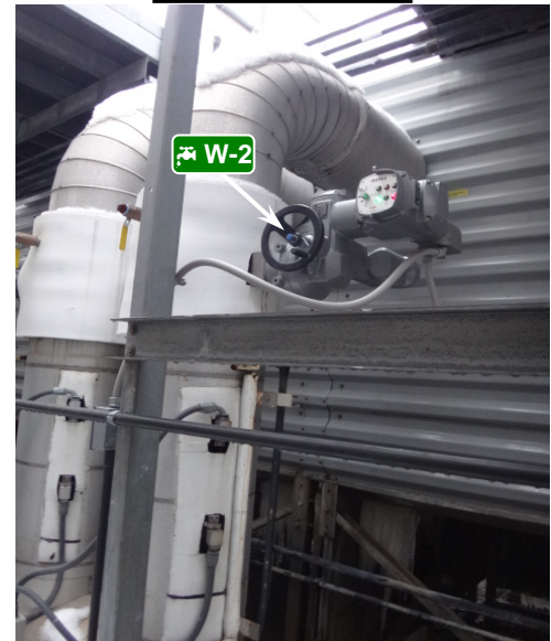
West Side View
