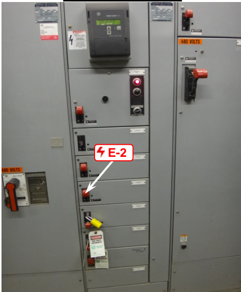
West Side View
