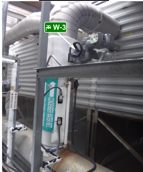
West Side View
