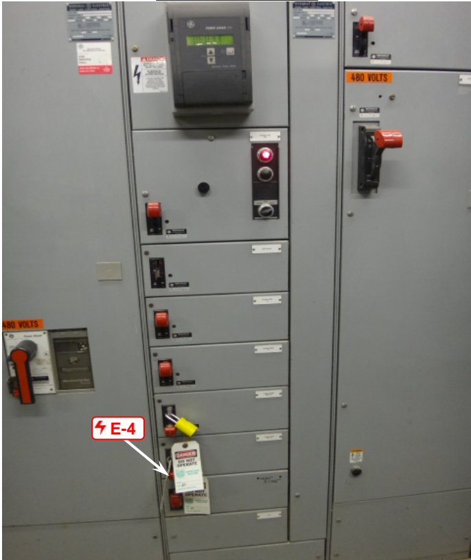
West Side View
