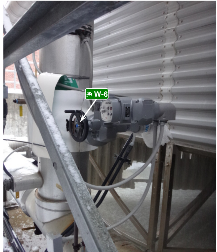
West Side View
