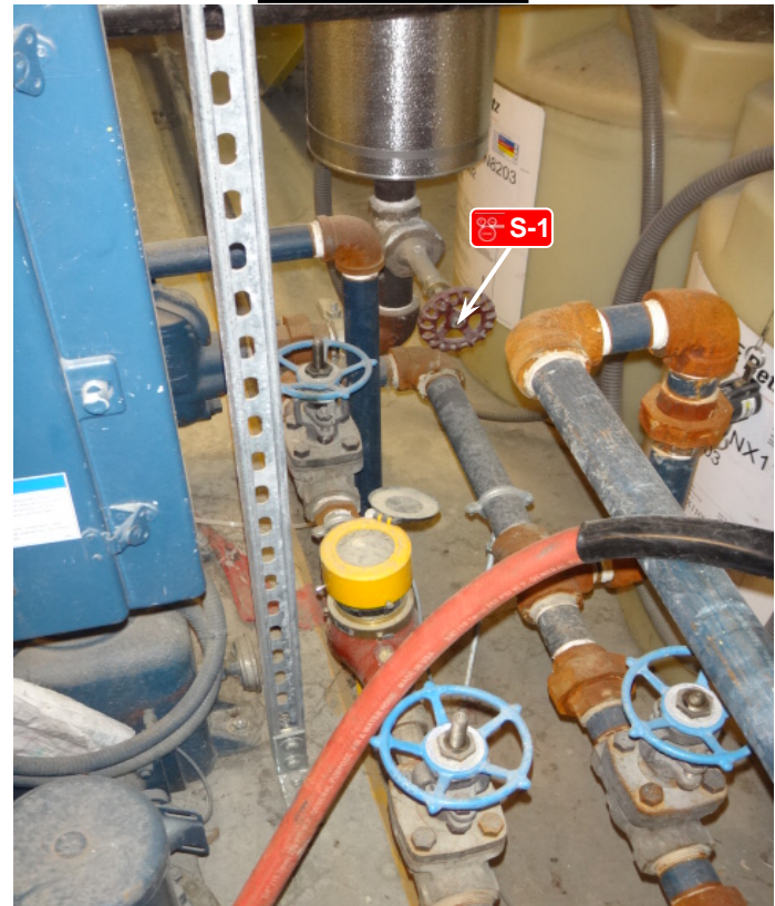
North Side View
