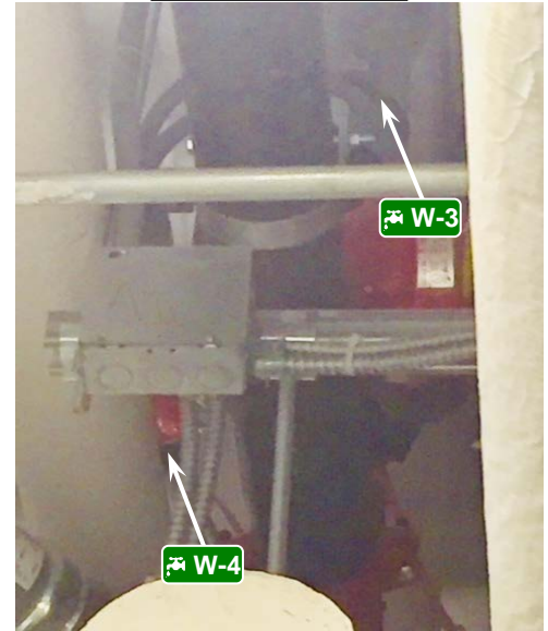
West Side View
