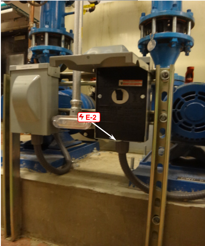
West Side View
