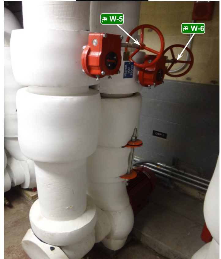
West Side View
