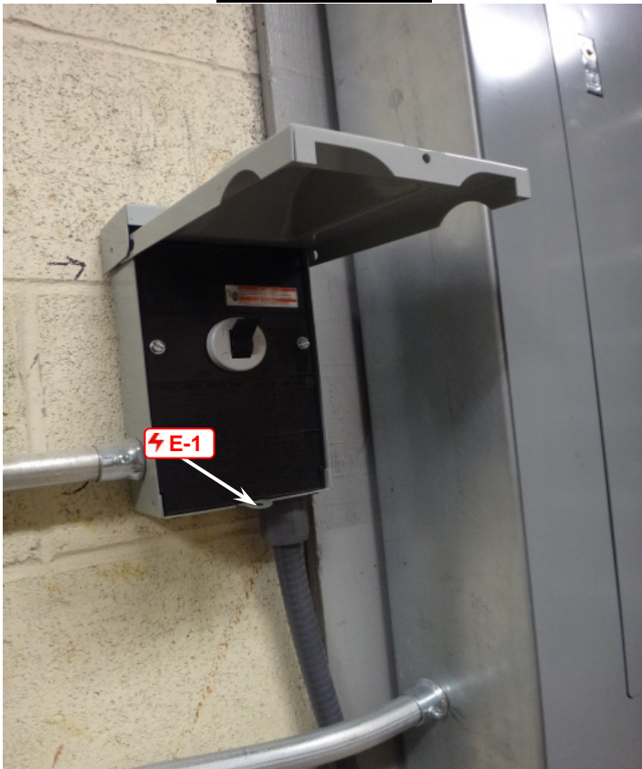
West Side View
