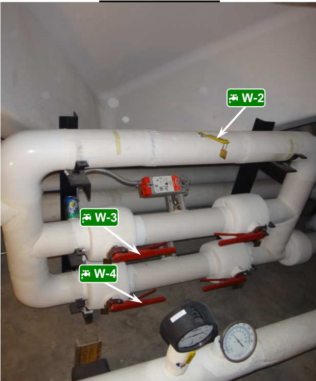
West Side View
