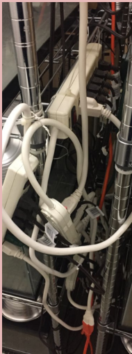
Long daisy chain: Three full power strips in series on an extension cord
